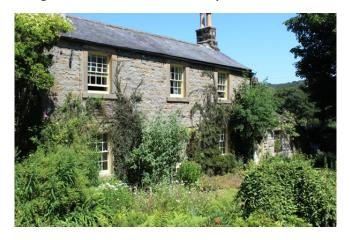
Outcrops of limestone provided quicklime for agricultural and building purposes. Most of the traditional building stock is constructed with an inner and outer face of sandstone set in a lime mortar with rubble-stone infill in the core of the wall.
